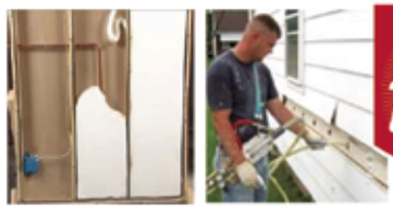
EMPTY, FILLING AND FILLED STUD CAVITY
